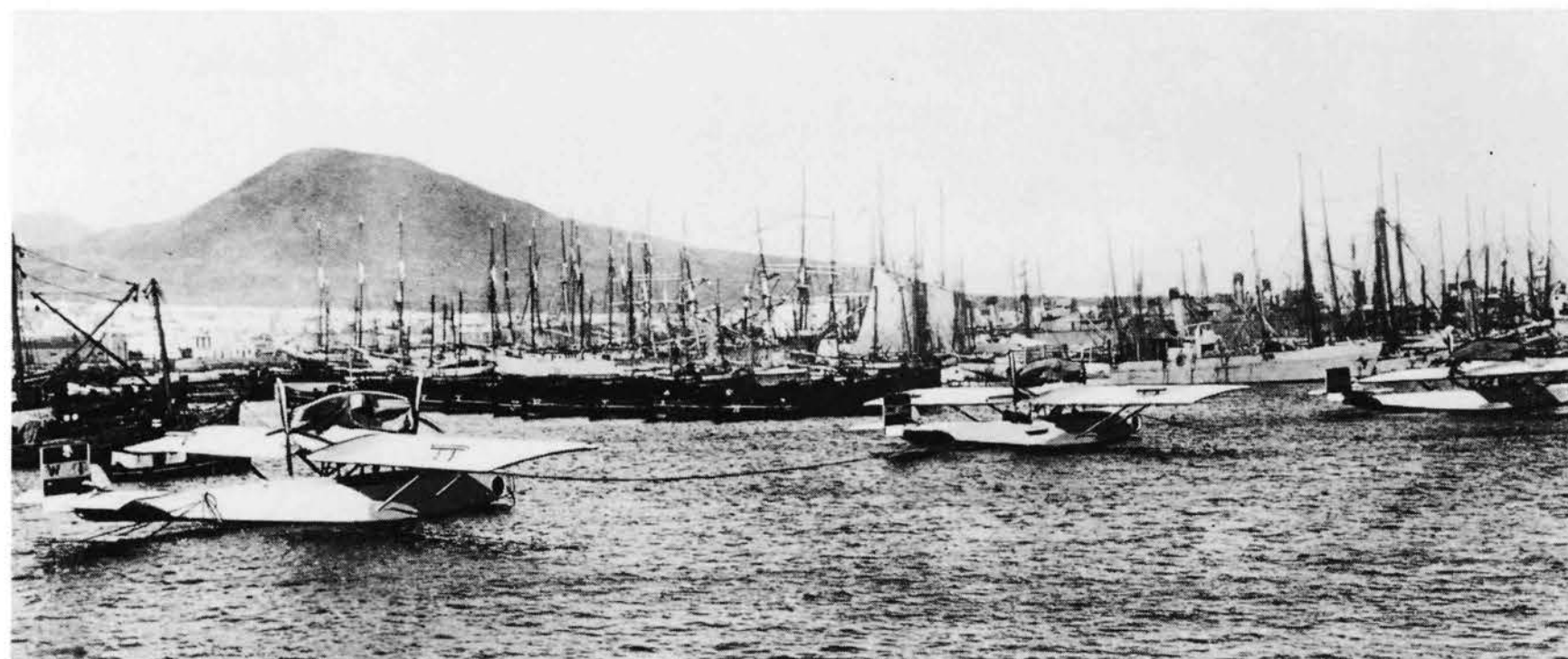
Above: Three CMASA-built Dornier Do J Wals of the Spanish Navy at anchor at an unidentified location, possibly Barcelona? The nearest aircraft is W-1, the others are unclear single-figure serials. All are wearing covers over their tandem-mounted engines. (via Harm Hazewinkel)
