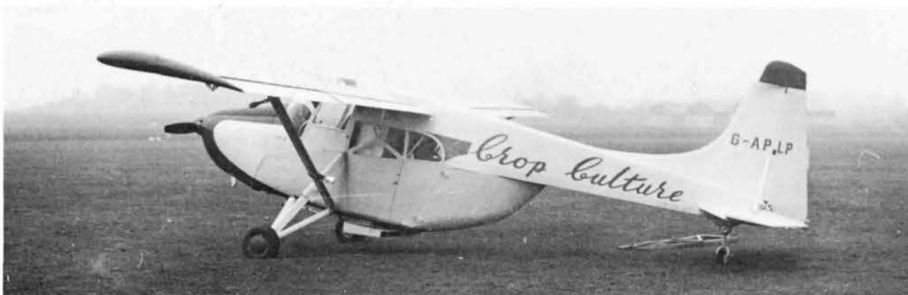
Left: G-APLP c/n 35 was used by Crop Culture of Bembridge after its CofA 31.3.58 and is seen with a duster venturi below the fuselage hopper, which is also visible through the cabin window. In 7.59 it reverted to Lancashire Aircraft at Blackpool but on 15.7.59 it force-landed on the beach, turned over and was submerged by the tide. (Aeroplane via JM)
