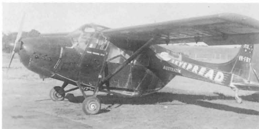
Left: G-APLP c/n 35 was used by Crop Culture of Bembridge after its CofA 31.3.58 and is seen with a duster venturi below the fuselage hopper, which is also visible through the cabin window. In 7.59 it reverted to Lancashire Aircraft at Blackpool but on 15.7.59 it force-landed on the beach, turned over and was submerged by the tide. (Aeroplane via JM)
